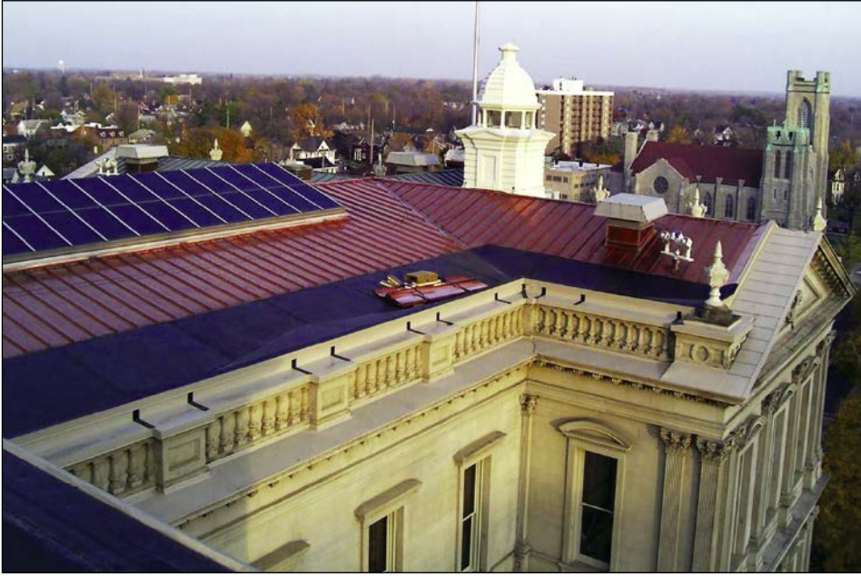
The sun's glow brightens the copper rooftop of Michigan's Capitol. The overall roofing plan called for installation of a new copper batten seam double lock system installed up to the ridge and a 90 mil, fully adhered Firestone EPDM roof on primed Dens deck in the valleys.
