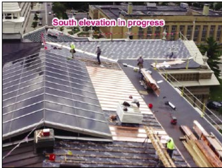
The work of CASS Sheet Metal and Bloom Roofing Systems is displayed in all its glory in this multi-directional panorama of copper and heavy-gauge rubber roofing.
